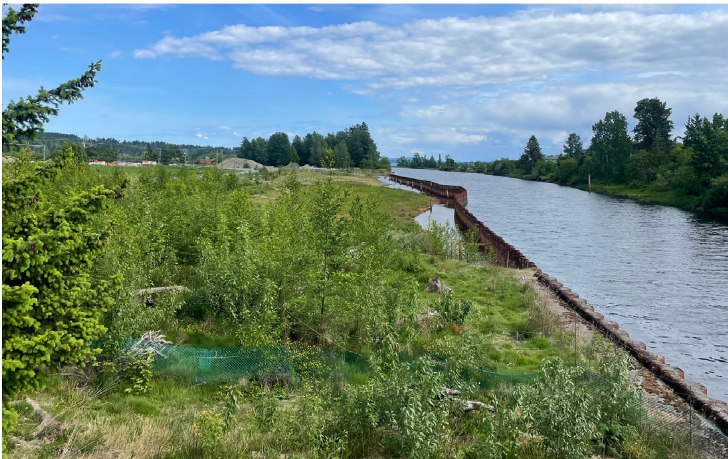
Our Coastal Region board has approved more than $1 million in the past six years to help purchase and restore a former sawmill site on the Courtenay River. The last panel of a steel retaining wall at Kus-kus-sum was removed in February 2026. The project is led by Project Watershed, in partnership with the K'ómoks First Nation and the City of Courtenay. 2026. Photo: C. Doucet
